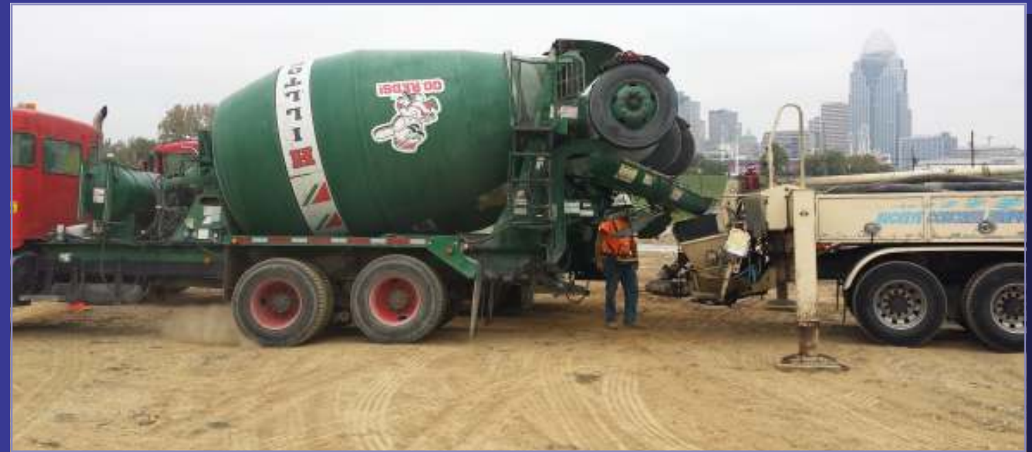
Below: A Hilltop Ready Mixed Truck fills the pump truck for the Roundabout operation
