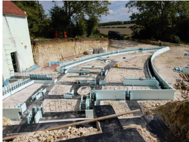
Above: The footprint of the house shows the first course of ICF forms have been placed. Below: The ICF forms are ideal for the curved structure and below grade construction.
