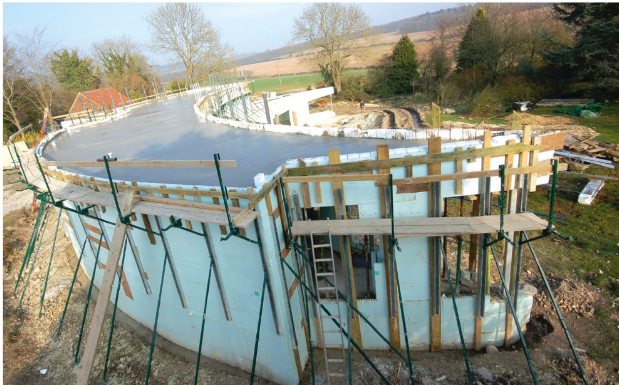
Above: The footprint of the house shows the first course of ICF forms have been placed. Below: The ICF forms are ideal for the curved structure and below grade construction.
