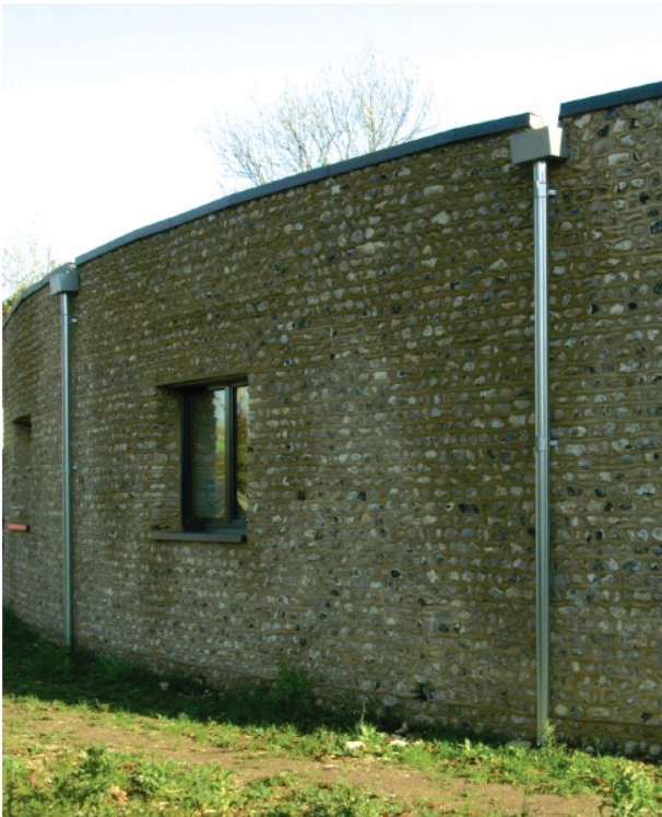
Salvaged traditional flint stone walls were incorporated into the new structure.
