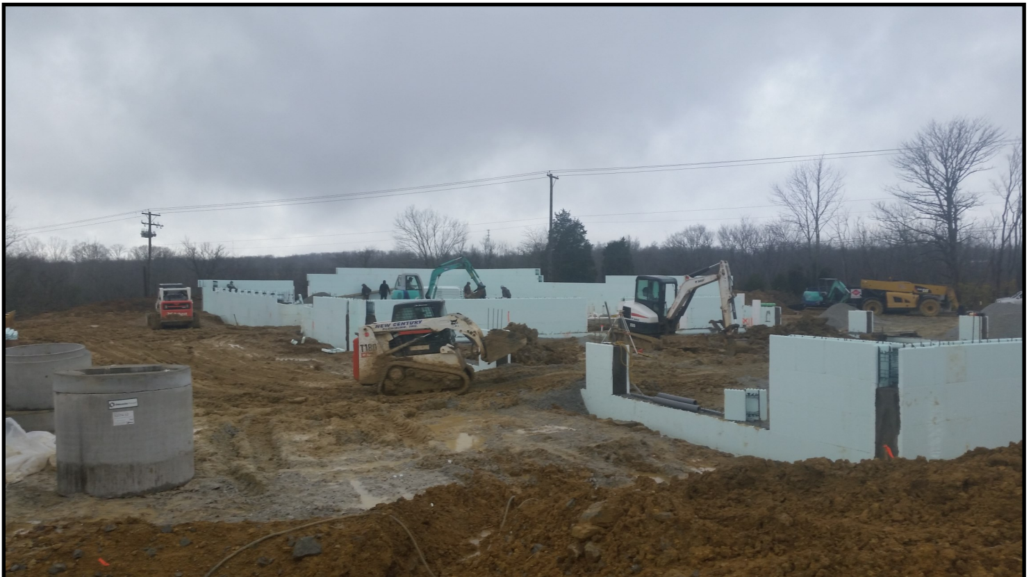
New EMS facility in Oldham County utilized ICF construction.
